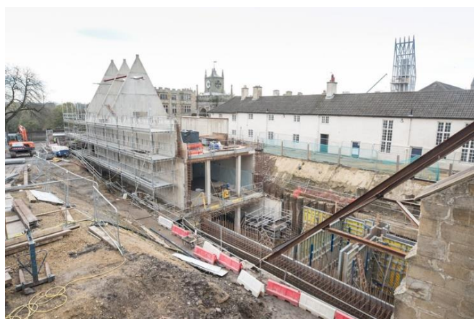
Above: Faith Museum under construction
