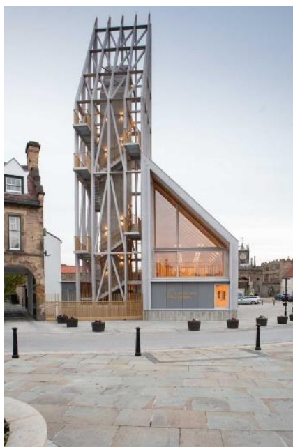
Auckland Tower © House of Hues
