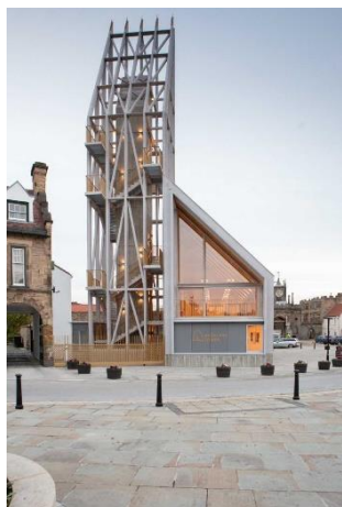
Auckland Tower © House of Hues
