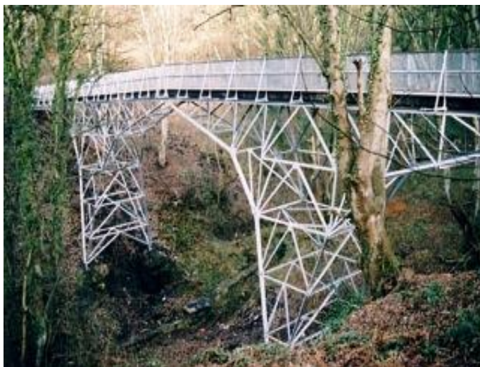
Figure 1 Silverlink Bridge - Gilesgate
