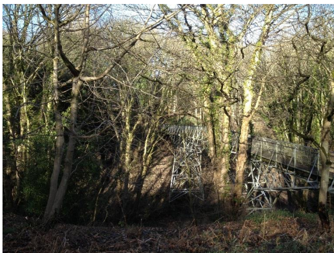
Figure 2 Silverlink Bridge as seen from SW
