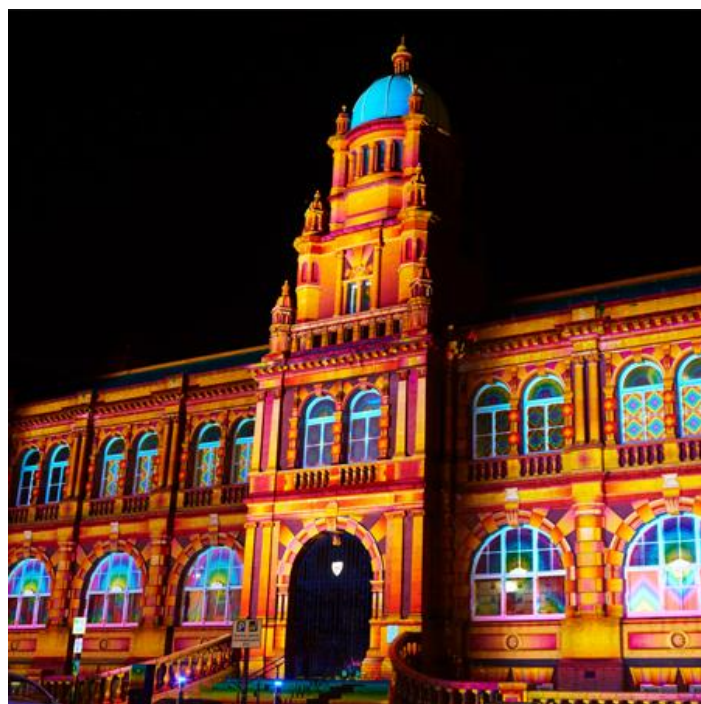
Photo: Durham County Council 2015
